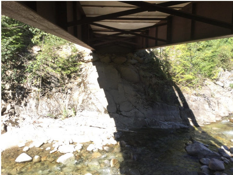
Right Bank Abutment when facing downstream
