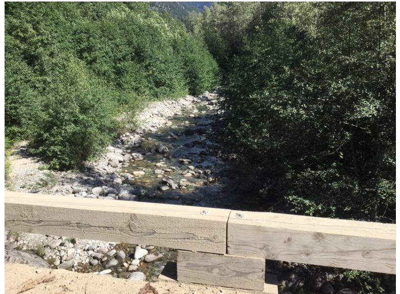
Upstream from Crossing
