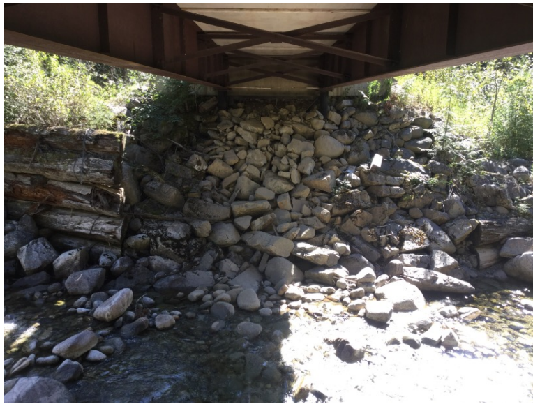
Left Bank Abutment when facing downstream
